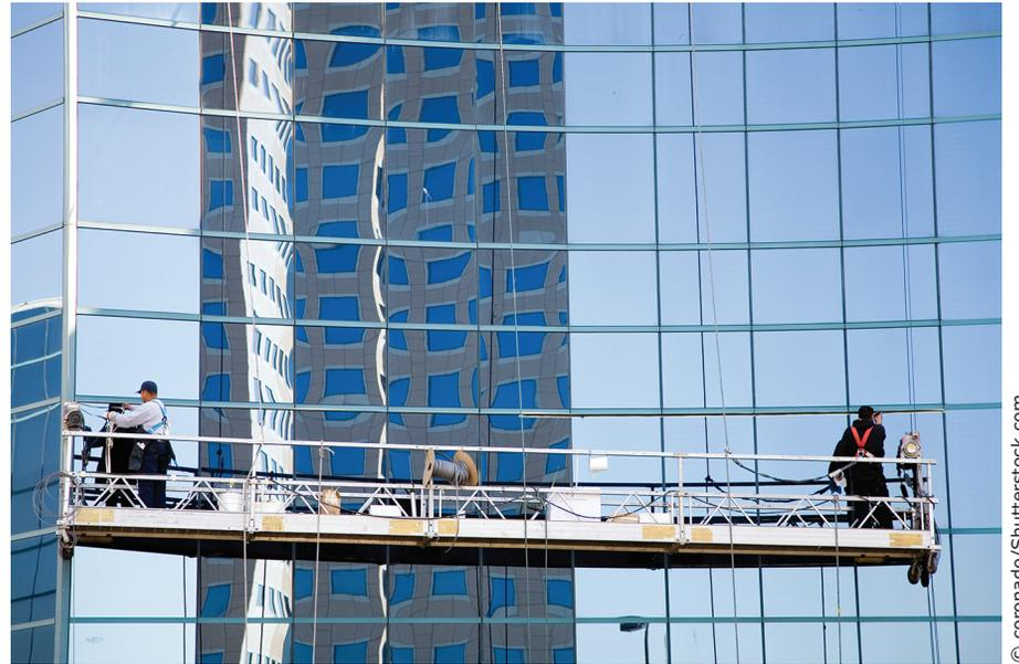
To do their job, skyscraper window washers needed new equipment. The Otis Elevator Company designed the first scaffold for skyscraper window washers. A scaffold is a platform that can be raised and lowered by cables attached to a machine on top of a building. Once the workers are finished, the machine on top of the building lowers them to the next level of windows below.
